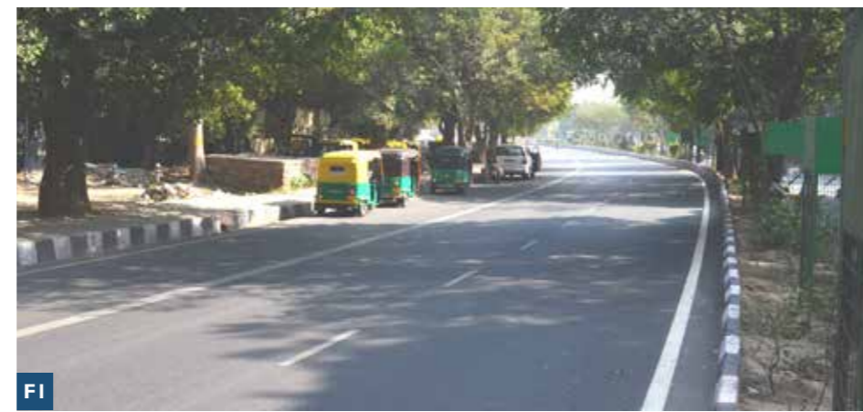
Road curving towards Malviya Nagar Metro station
