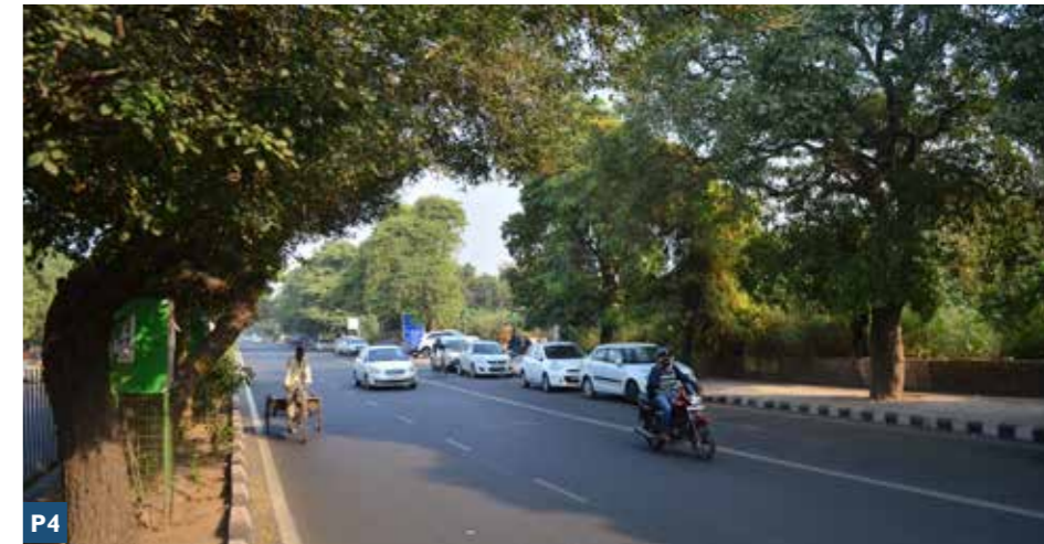
Satpula Drain along the carriageway of Press Enclave Marg (opposite Satpula Lake Park)
